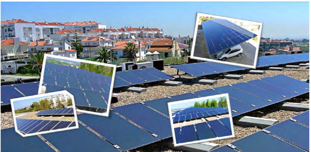
55 kW PV power station installed in FCT-UNL campus using a-Si:H solar cells technology implemented by CEMOP+CENIMAT and transferred to Solar Plus, 2013.
